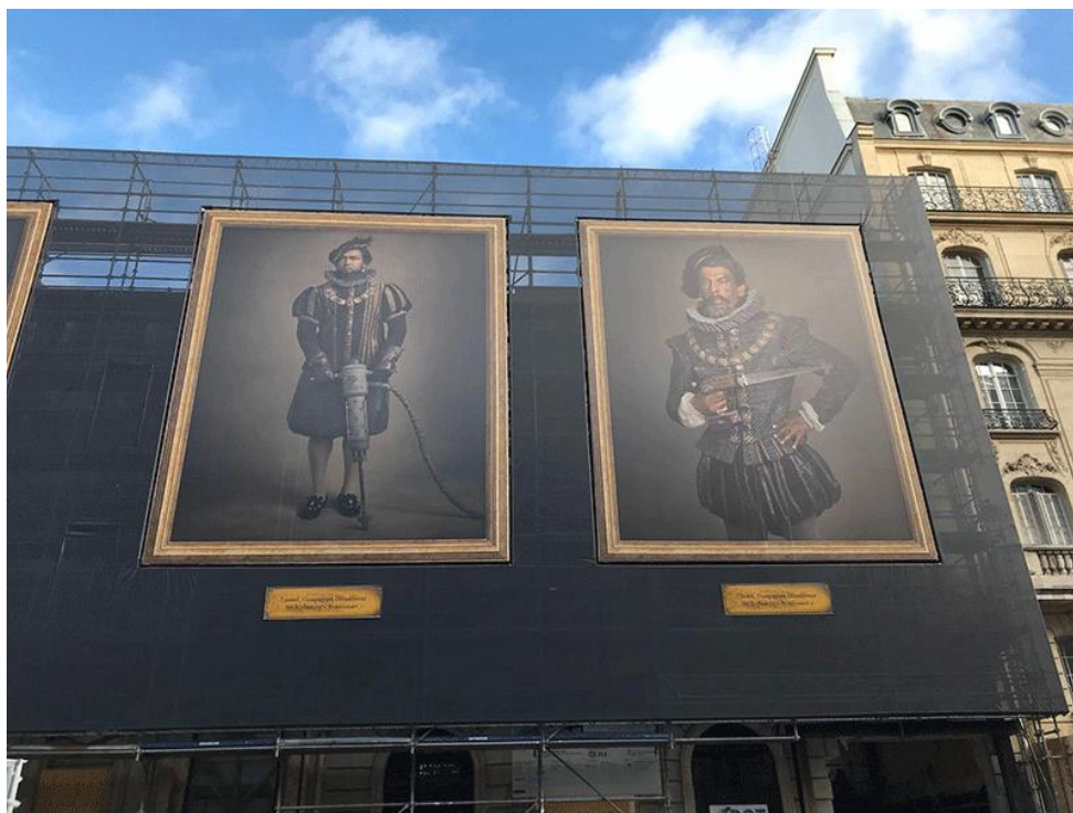
The scaffolding on rue François 1er.
